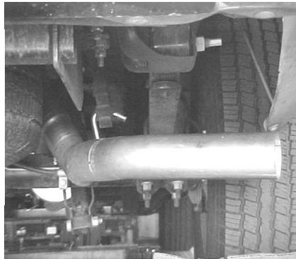
INSTALL TURNOUT PIPE #D INTO OVERAXLE TAILPIPE USING CLAMP# F. ROTATE EXIT PIPE UNTIL IT IS AT THE CORRECT ANGLE FOR YOUR TRUCK.
